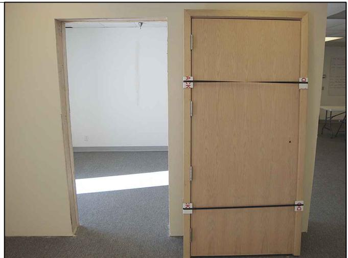
**VERY IMPORTANT (Floor Preparation):** Ensure that the floor under the door slab is flat and level. You may install a flat, level, and smooth threshold. If the existing floor is not flat, level, and smooth-the bottom door seal will not perform properly. **DO NOT** raise the hinge side of the jamb off of the floor. The factory undercut of the door is set to the proper height.
